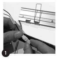
Cut 12-13mm (0.47-0.51") wide slot to required length. Bring through power feed and make connection to GROOVE In.
